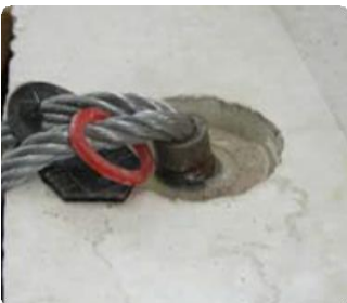
Wire slings bent over!
